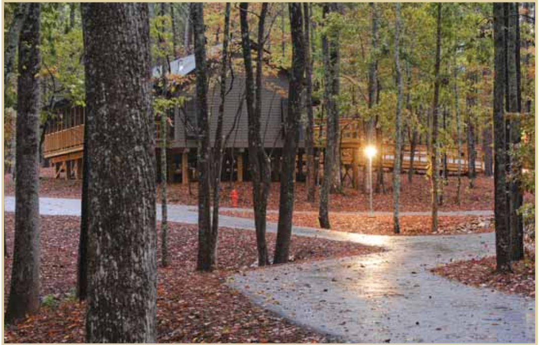
The cabins and conference center are nestled among the trees on the 16-acre site donated by Ben and Luanne Russell and Russell Lands. Harbor Lodge is an extension of the existing facilities on the Lake Martin campus.
